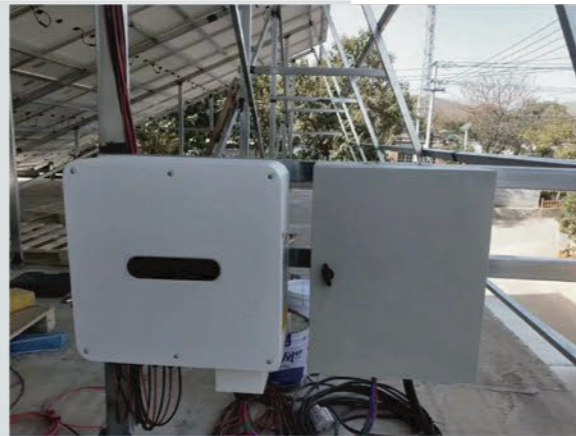
Residential PV Project in China
